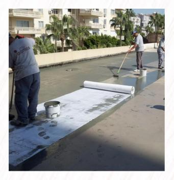
At wet on dry waterproofing systems, it is only possible to apply the top coat after the base coat is cured. The waiting time period between the coats causes poor adhesion between each other regardless of the final thickness and number of coats. Each thin coat will act independently and this risky phenomenon for the entire performance of the system, may lead to delamination between the coats.
